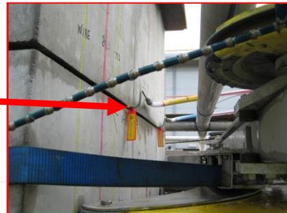
Fig 2: PowerPads within cut gap
